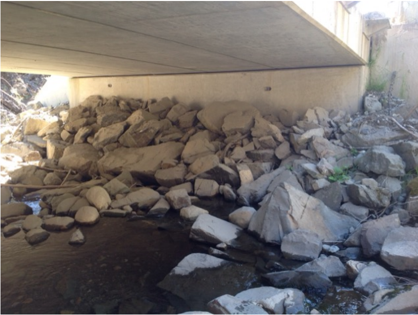
Right Bank Abutment when facing downstream
