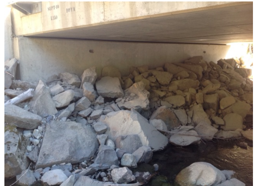
Left Bank Abutment when facing downstream
